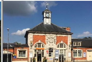
Hatch End Station
